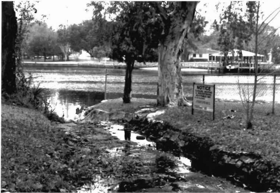
Figure 42. The end of this road abuts the river. The sign states that it may be vacated as a public way. This action will preclude using the land as a catchment for stormwater, "pocket park", or habitat patch. Note the runoff draining from the street into the river. With vacating, not only will the potential for improvement be lost, but drainage will probably be "improved" by installing a culvert.
