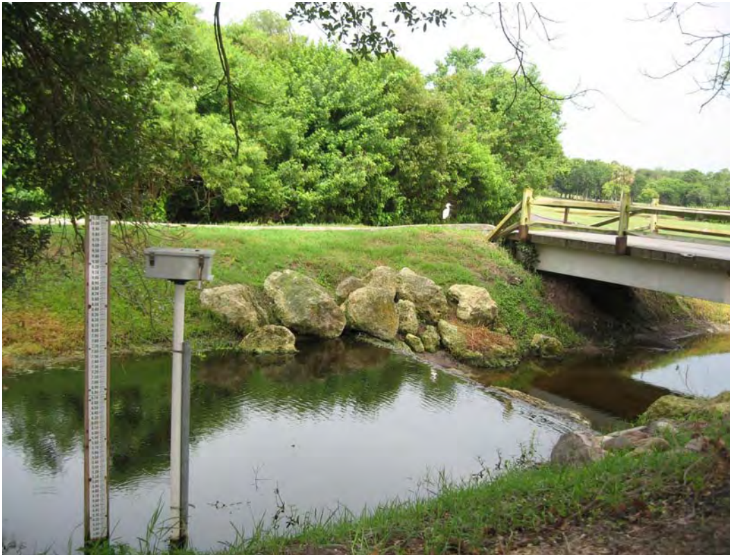
a. Gauging Station Upstream from the Horizontal Weir
