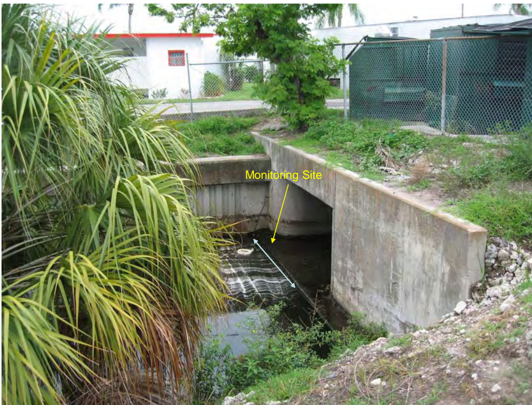
b. Box Culvert Discharge Monitoring Site
