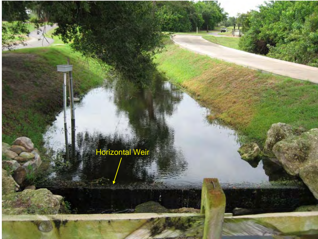
b. Horizontal Weir Structure
